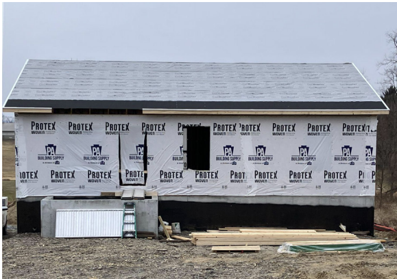
B&H Blitz Build on Richard Ave - A house in just 5 days!
